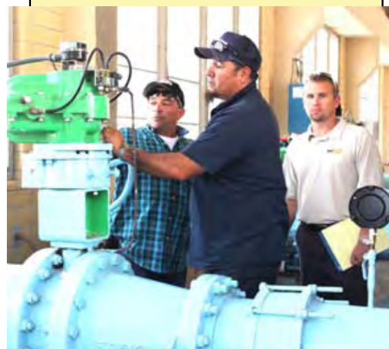
A hands-on workshop, presented by the EPA and Texas Manufacturing Assistance Center, guided water system managers and technicians in measuring the amperage, voltage and other data related to water pump motors. Specialized software uses the data to determine how to operate the water pumps most efficiently. (VBR)
