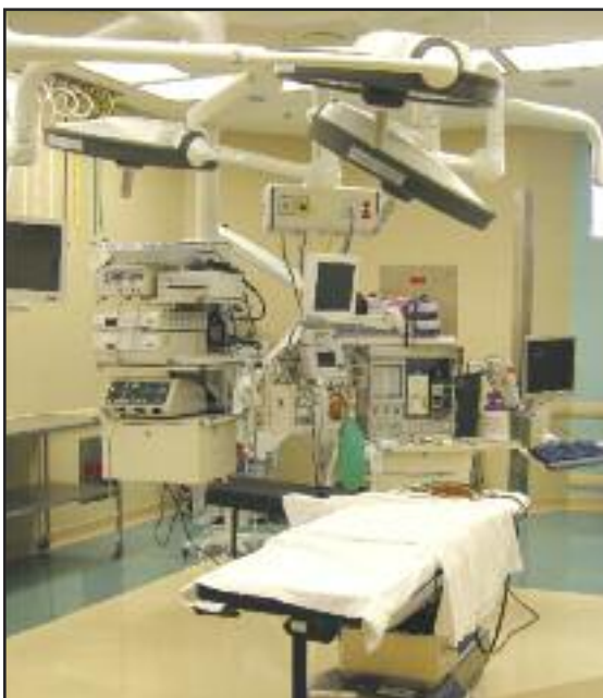
The new operating suites have equipment on booms overhead, freeing floor space for surgeons, nurses and technicians. (courtesy)
