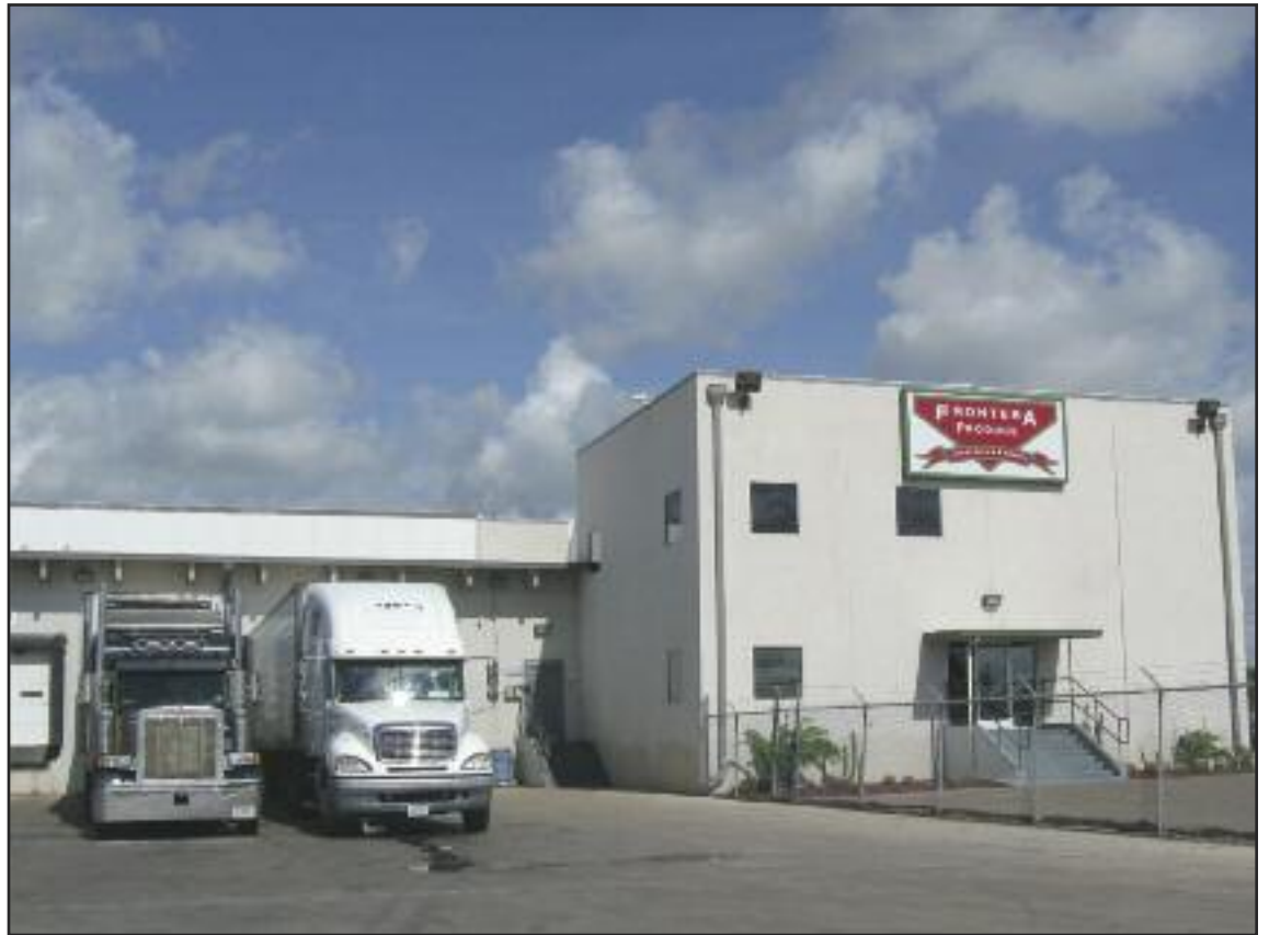
At this time of year, Frontera Produce's Edinburg facility does more cross-shipping than packing. (Mattei)
