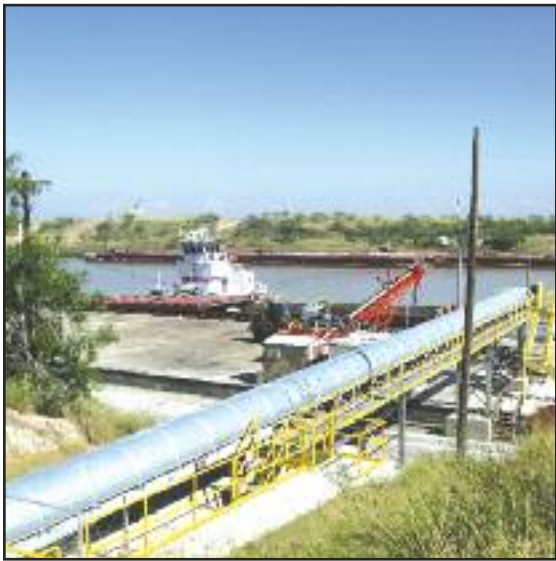
Raw sugar travels by conveyor from the Sam Sparks Sugar Warehouse to a waiting barge at the Port of Harlingen's main dock.. (Mattei)
