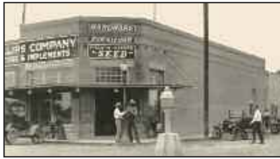
Jackson Street intersection as it looked one hundred years ago. (courtesy)
