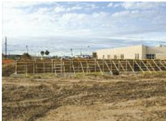
Edinburg HS Performing Arts Facility currently under construction. (John Faulk)
