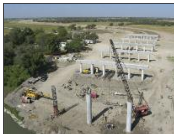
Roadway section under construction. (courtesy)
