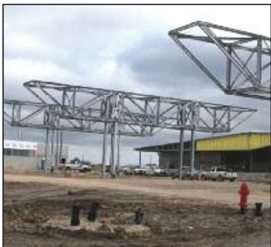
Construction near the Donna bridge. (courtesy)
