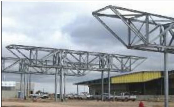
A new bridge for Donna / pgs. 6 - 7
