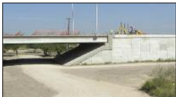
Bridge overpass nears completion. (courtesy)
