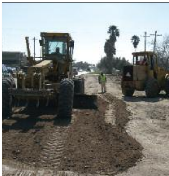
Construction zones work on expanding Valley roadways. (Kevin Knoch)
