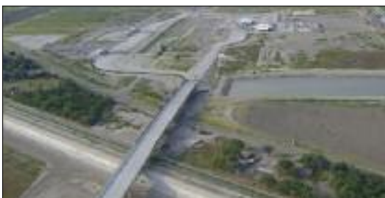
Anzalduas Bridge nearing completion, vital access for Valley. / pg. 10-11
