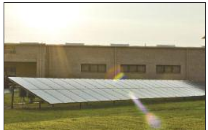
New solar energy panels now provide electric power for the Autobody Collision Technology Building at TSTC.
